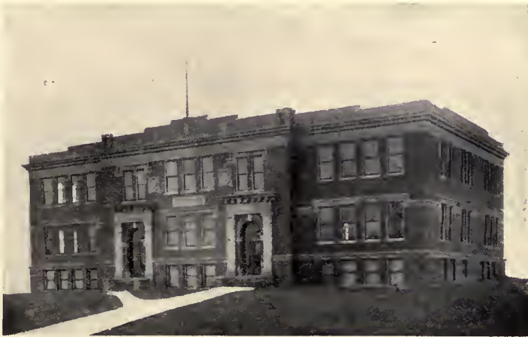
THE LAWRENCEVILLE, LAWRENCE COUNTY, HIGH SCHOOL
